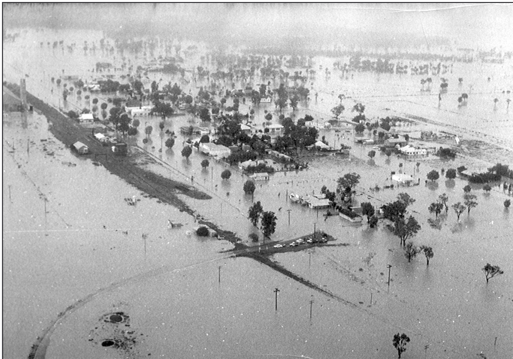
Figure 6 - Photograph of Garah in 1976 Flood (Looking South-West)
