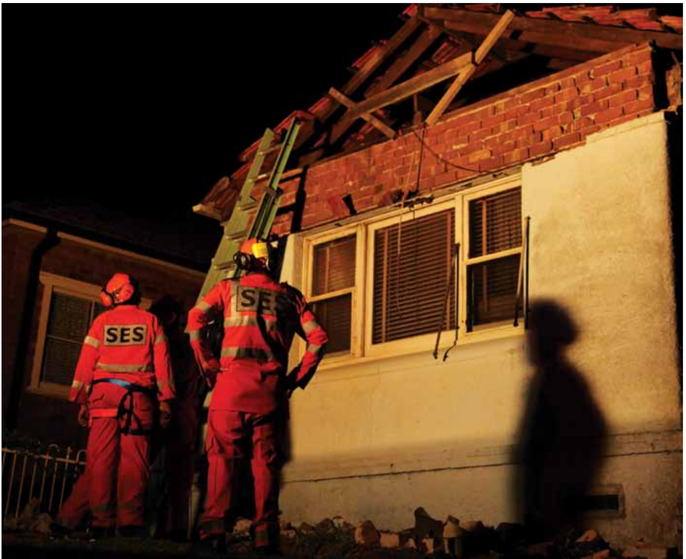
Canterbury Unit members respond after strong winds cause damage to a house, Beverly Hills NSW
