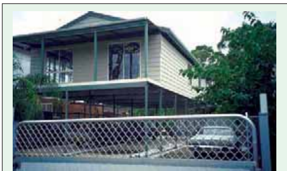
Figure 49 Raised house construction provides a high level of protection
