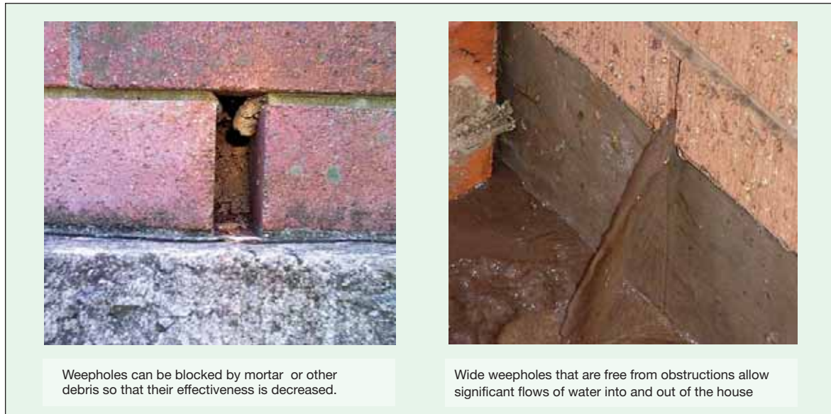
Figure 93 Careful detailing of weepholes to avoid problems
