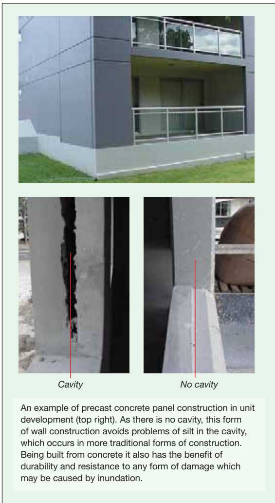
Figure 58 The advantages of concrete panel housing
