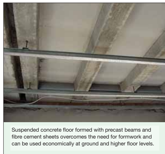
Figure 74 Suspended concrete floor
