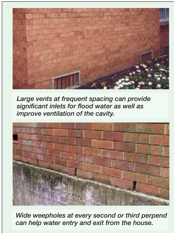
Figure 30 Water inlets in external brick cladding
