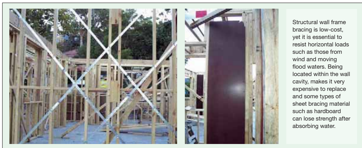
Figure 85 Durable frame bracing
