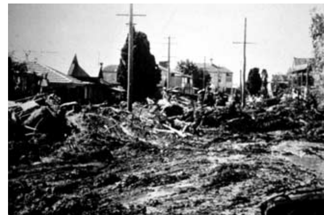
Maitland in the 1955 flood – flood debris
